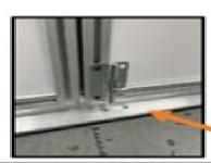
Bottom barrel lock secures the smaller door section when unused.
