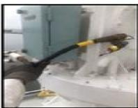
Connect both pressure hoses on both suction and pressure line respective to its colour band
