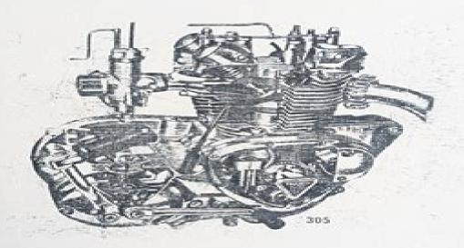
UNIT CONSTRUCTION 350 c.c. and 500 c.c. TWINS
